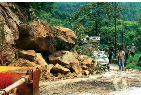
Landslide at Hati Surey (NH31A) - Aug2008.
